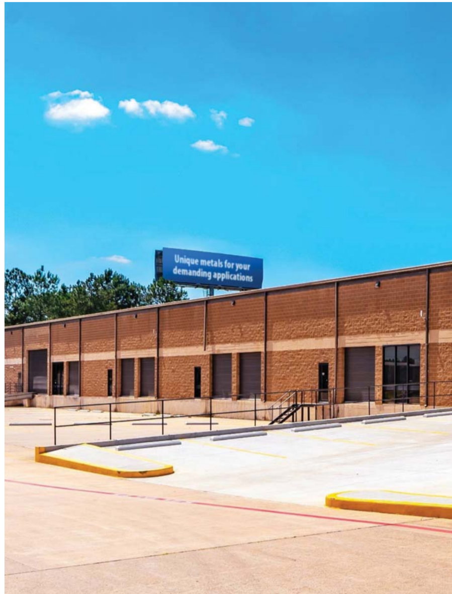
Langley Alloys' new facility with an area in excess of 30,000 sq. ft., which is double the size of
